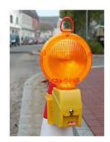
All street and road works on roads with a speed limit of 40 mph or more **must** have warning lights illuminated in poor visibility or during the hours of darkness. If your risk assessment requires it, warning lights should also be used on lower-speed roads.
