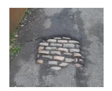
All is not what it appears!!! On occasion we excavate in a carriageway or footway with a bituminous surface to find that just underneath there are cobbles, sets or other modular materials which formed the original surface which has over time been overlaid with HRA or DBM material.
